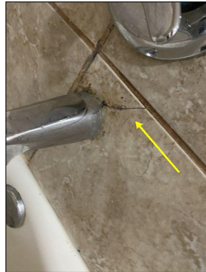
Broken tile observed.
