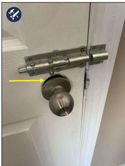
Door lock missing or loose. Recommend repair or replacement by qualified contractor.
