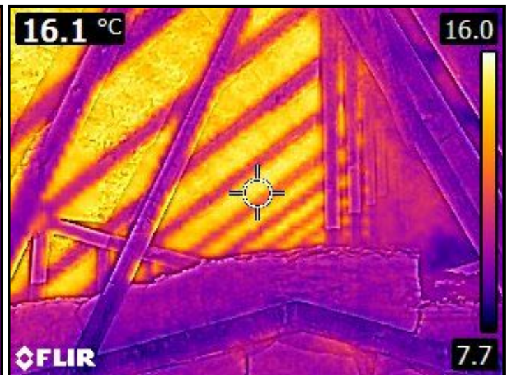
Appeared functional at time of inspection. No deficiencies observed.
