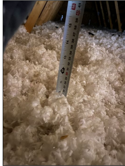
Insulation appears adequate.
