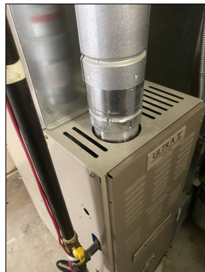
Operational/Functional. No major concern at the time of inspection.
