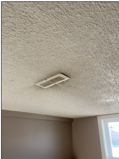
The return air supply system appears to be functional.
