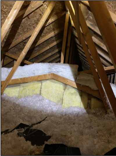
Insulation appears adequate.
