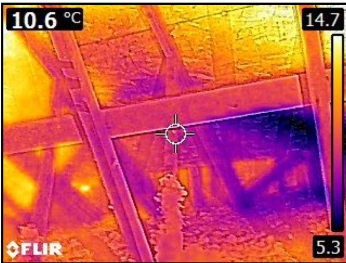
Insulation appears adequate.
