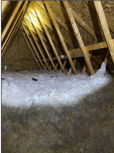
Appears functional at the time of inspection.
