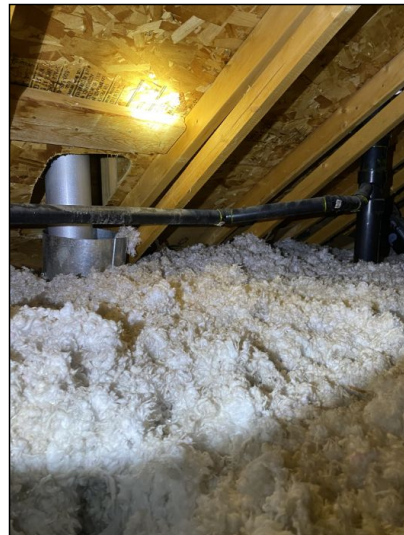
Appears functional at the time of inspection.
