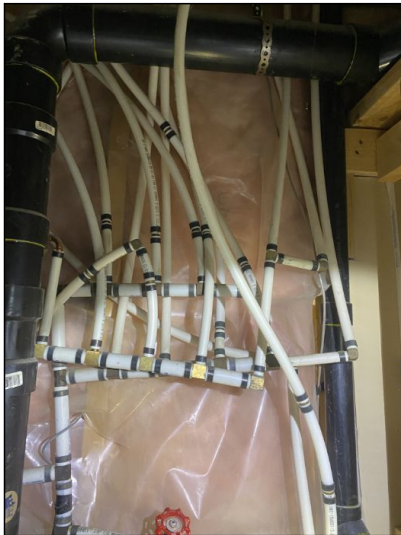
Functional at the time of inspection.
