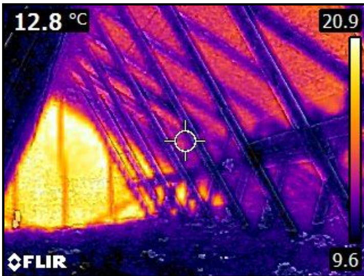
Appears functional at the time of inspection.
