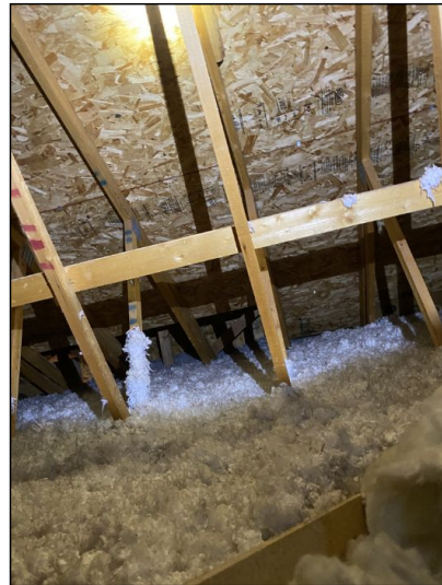
Appeared functional at time of inspection. No deficiencies observed.
