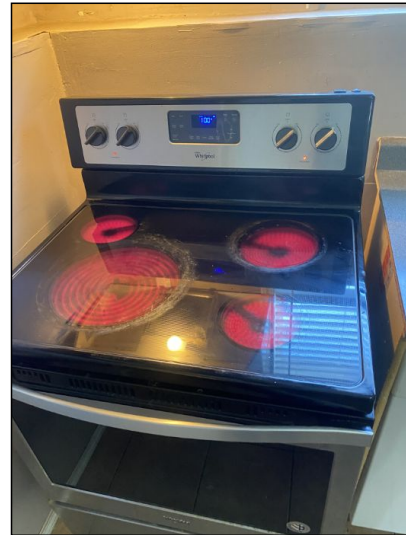
Operational/Functional at the time of inspection. No deficiencies observed. Cosmetic damages are not included in the inspection report.
