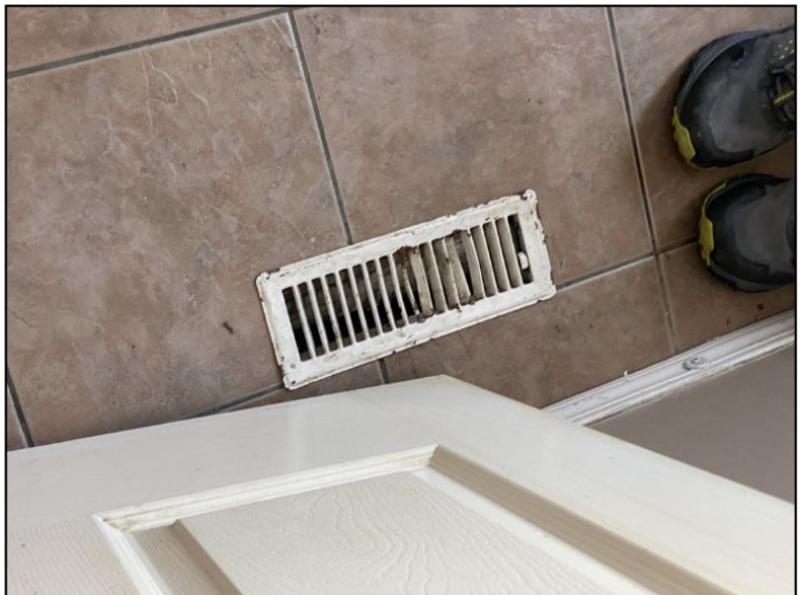
The return air supply system appears to be functional.
