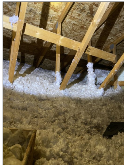
Insulation appears adequate.
