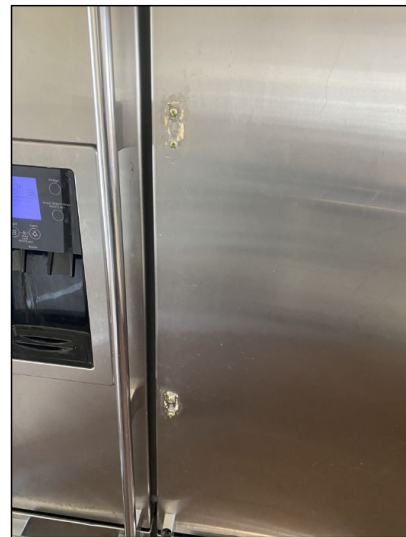
Water and ice dispenser is inoperable and the door handle observed missing.
