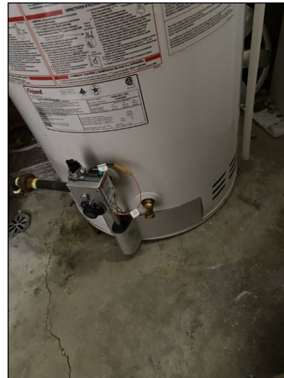
The water heater base is functional.
